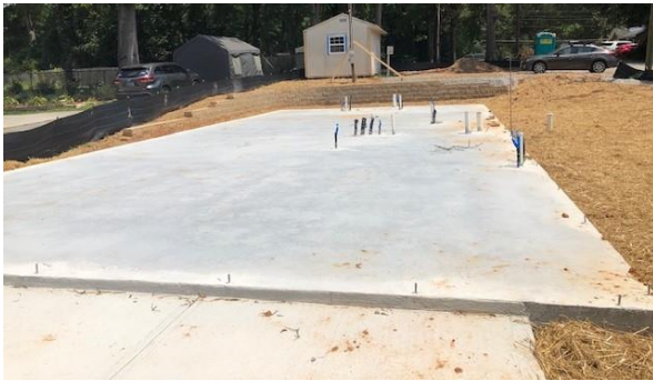
The build has a slab & retaining wall.
